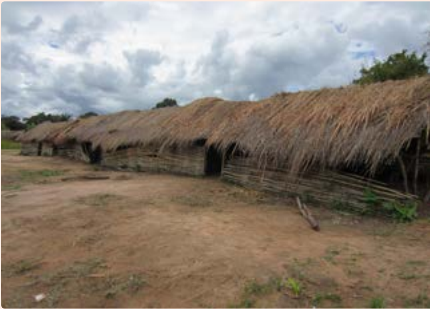
PICTURE 7: SCHOOL EP F, TEMPORARY BUILDING CONSTRUCTED USING LOCALLY AVAILABLE RESOURCES
