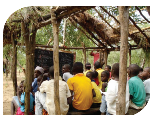
2. Stick and thatch construction classroom – Caimbambo
