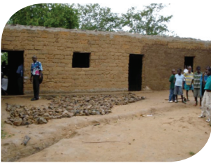
4. School constructed of typical mud 'Adobe' bricks – Caimbambo
