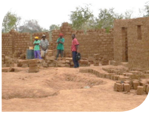
5. School building under construction using 'Adobe' mud bricks – Caimbambo
